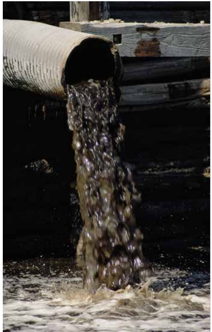
Sewage treatment plant
